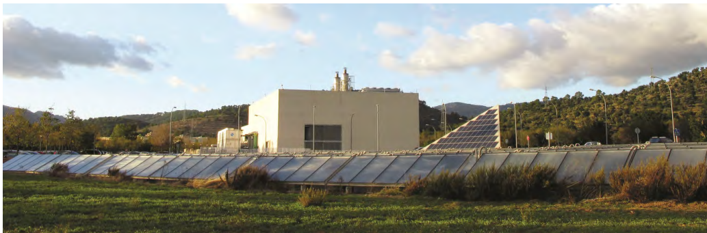
Figure 1.2: Frontal view of Parc Bit power plant
