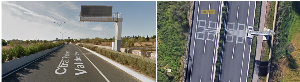
Figure 2.5: Vehicle Loop Detector on the road. Image from Google Maps
