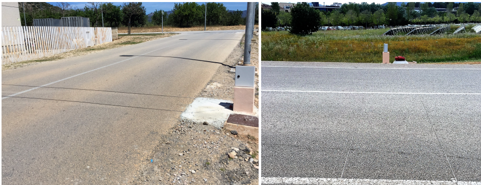
Figure 5.4: Node S4 in E2 (right) and node S7 in E4 (left). The tubes are laid perpendicular to the road's direction.
