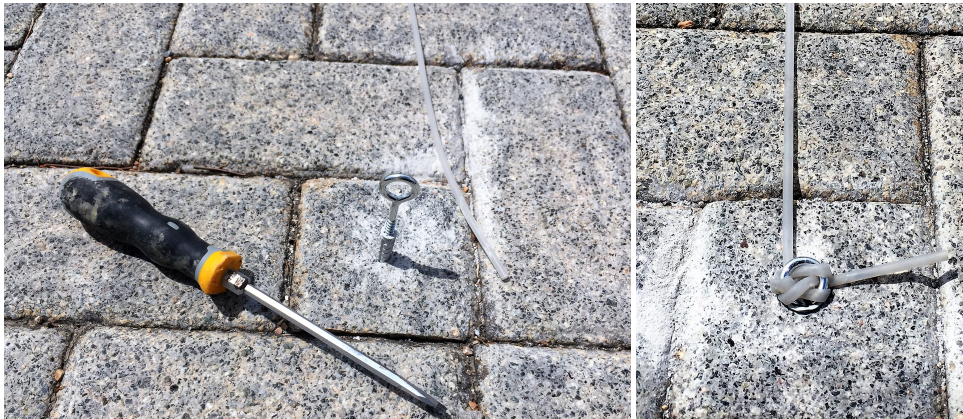
Figure 5.7: After doing a hole in the pavement, expansion anchor and the screw are inserted. Screw inserted and tube fixed.
