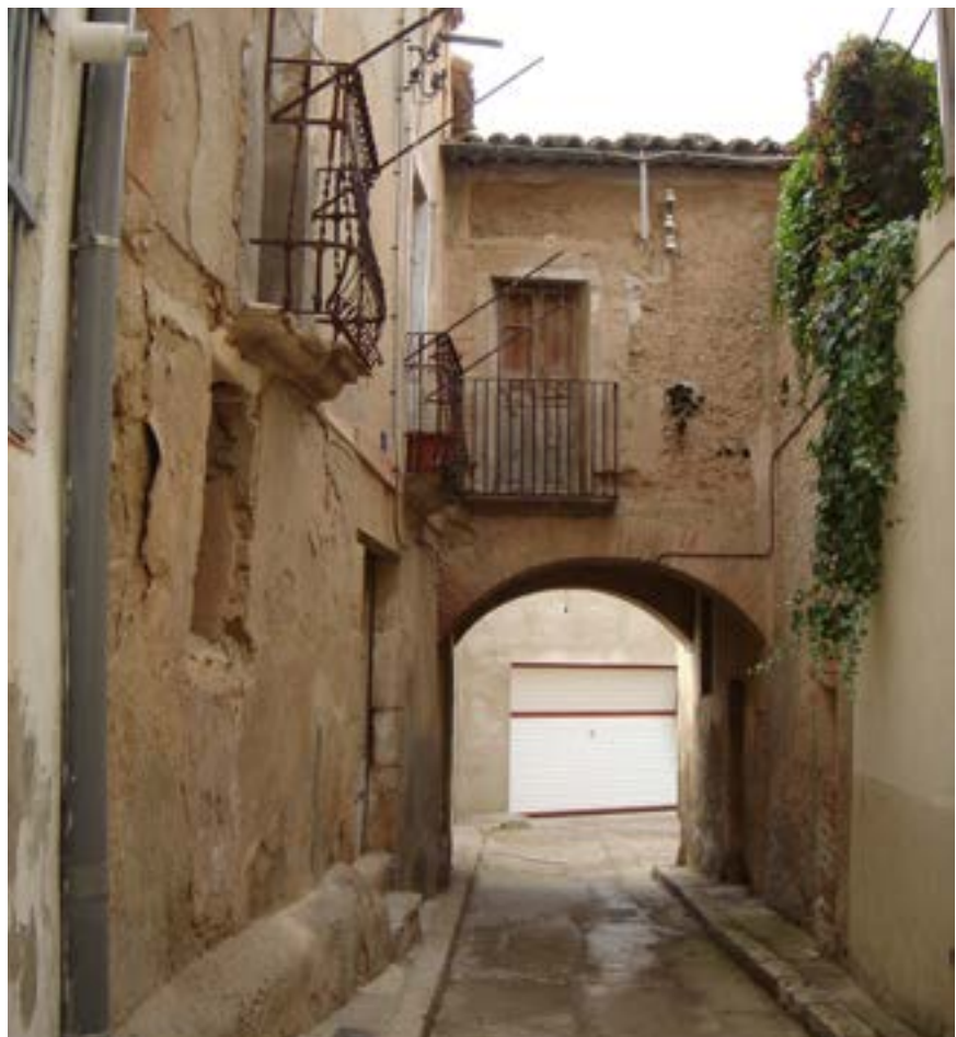
Carrer de Linyola (Pla d'Urgell), with an early 19th century house built with adobe. Author: Adriana Salvat Torregrosa.
