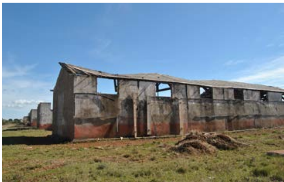
Part of the exterior of the Ribesaltes remains. ENRS
