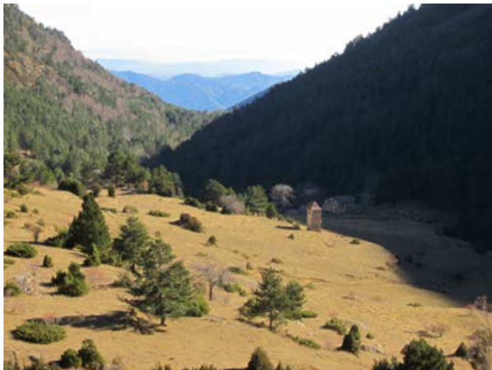
View of the Peguera valley, showing an old electricity pylon and the Cantina in an advanced state of disrepair (2013). FERRAN PONS
