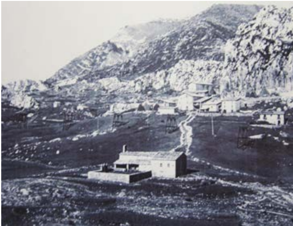
Panoramic image of Peguera, featuring the remains of the pylons that carried the cable car, allowing the transportation of coal extracted from the mines throughout the Peguera valley (undated photograph; mid-20 th century). PERSONAL ARCHIVE OF A RELATIVE OF EL PEGUERA
