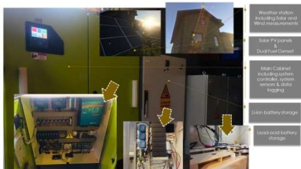
Figure 9 OHRES in Canada household case-study - System on ground commissioning
