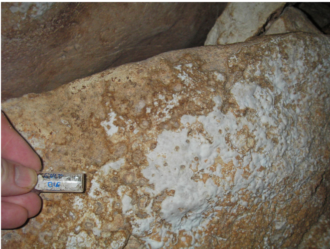
Fig. 12. Gypsum blisters covering a fallen boulder located in a well-ventilated area that is affected by outside air flows.
