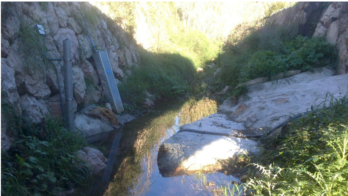
Fig. 3. Gauging section of the Sa Murtera station.
